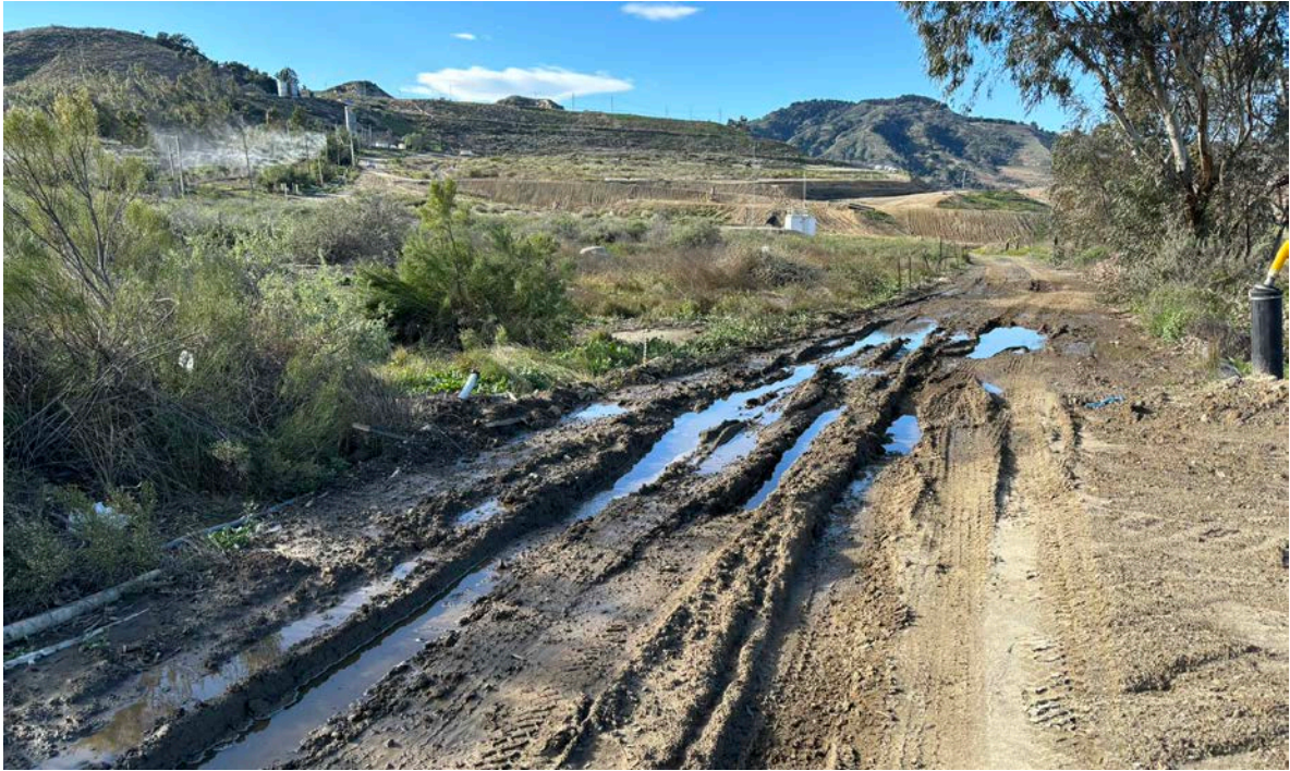
Maintenance access Road weathering on north side of Deck C
