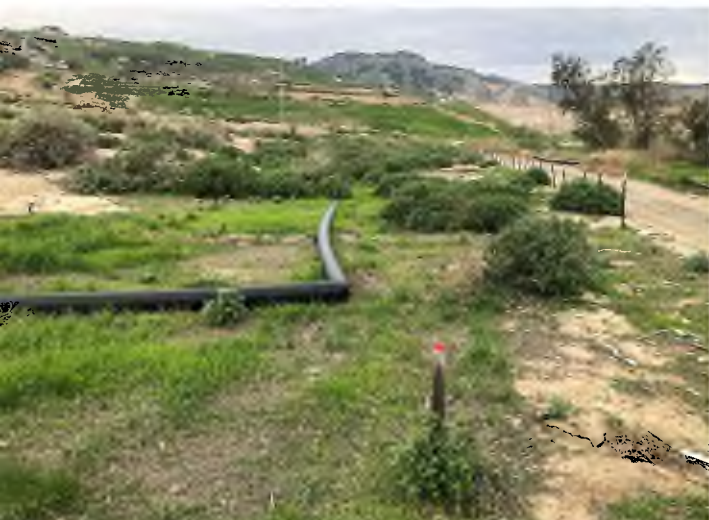
Photo Station #8 - December 2022 (West)
