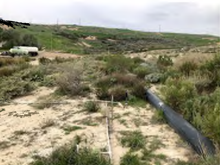
Photo Station #7 - December 2022 (West)
