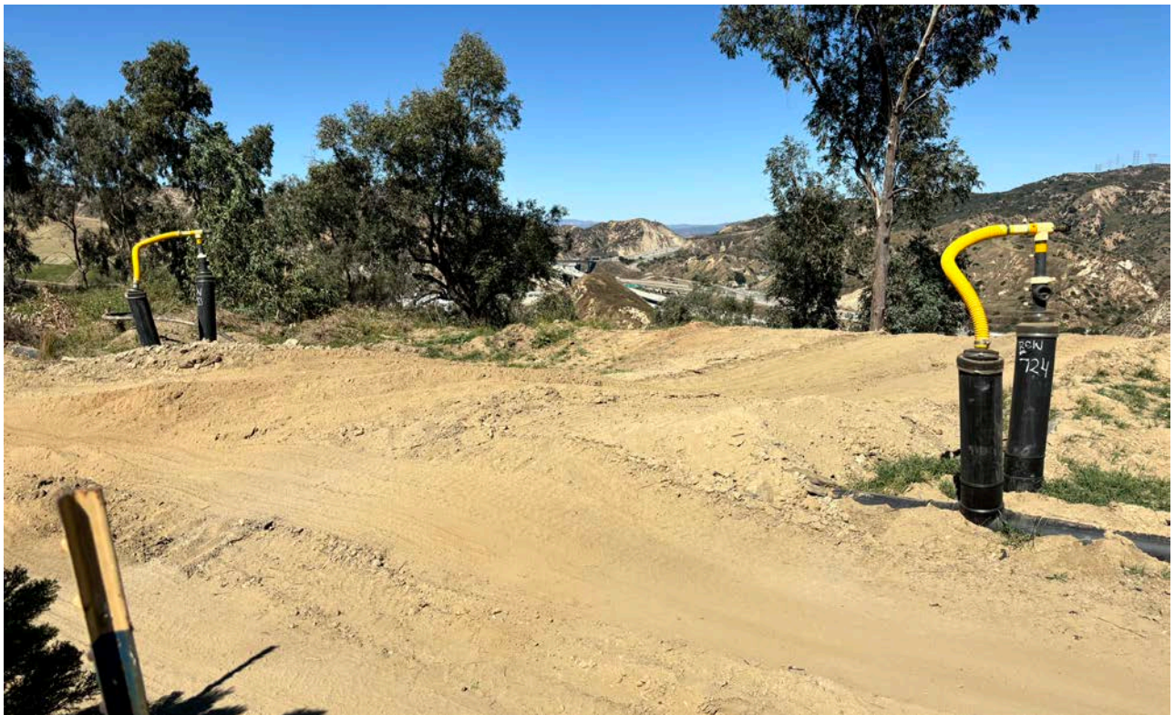
Recently graded areas surrounding Deck C
