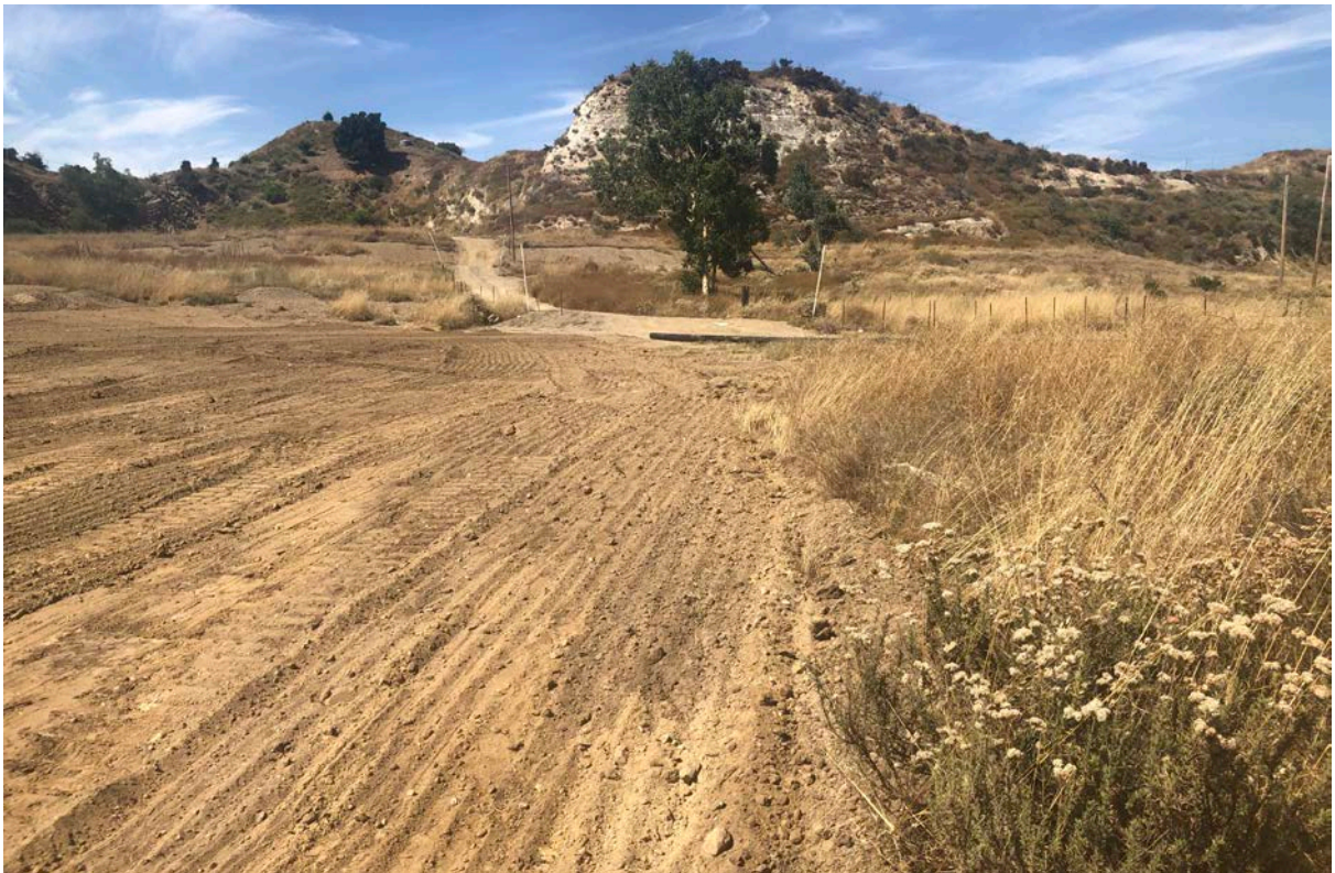
New grading at Deck A (view looking south)
