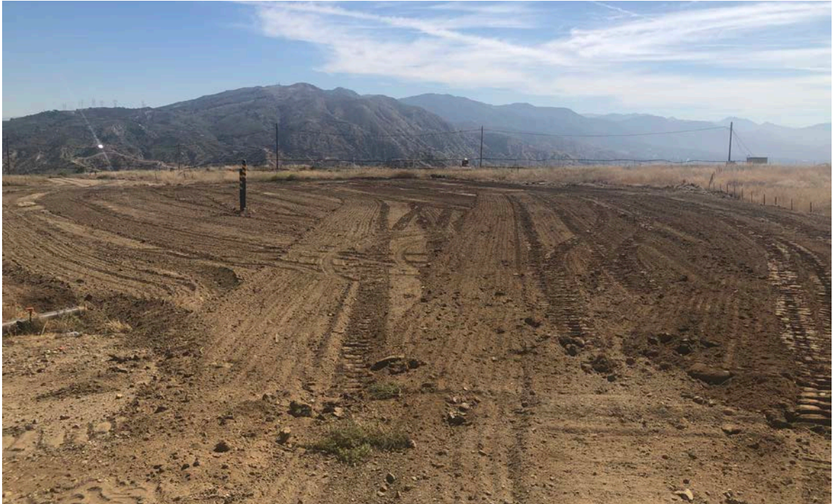
New grading at Deck A (view looking east)
