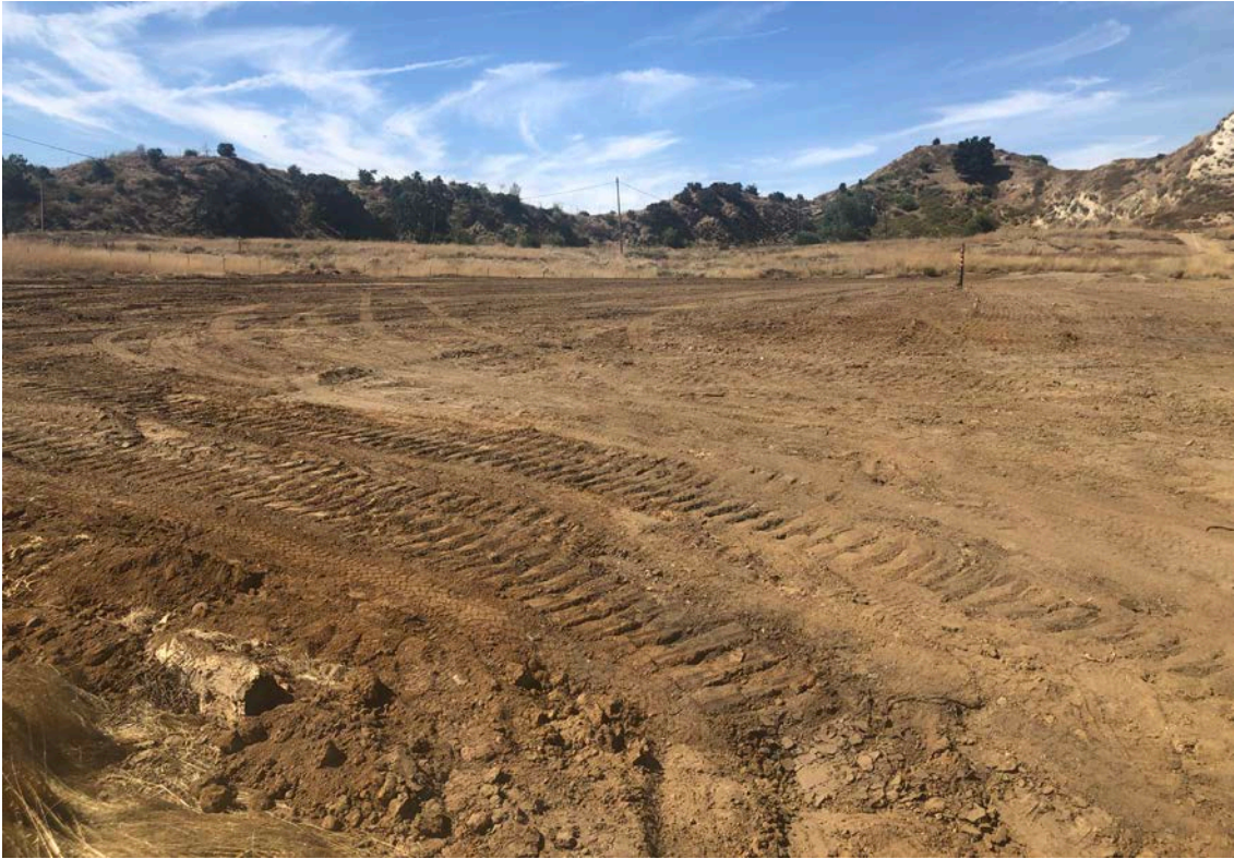
New grading at Deck A to correct drainage issues
