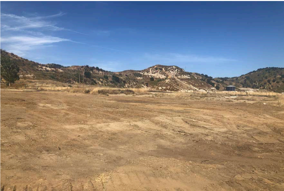
New grading at Deck A to correct drainage issues
