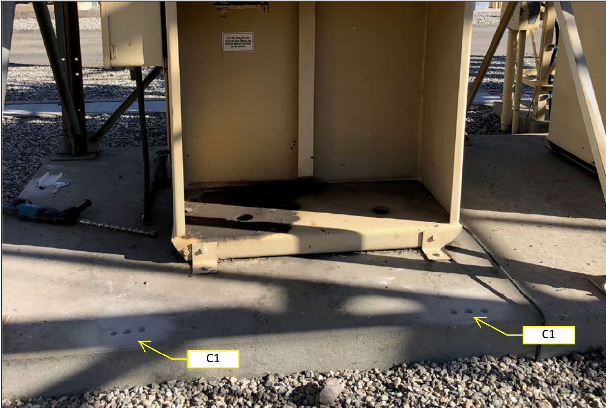
PHOTO 3: COMPOSITE CONCRETE SAMPLE LOCATION C1 DOWNEY SUBSTATION, DOWNEY, CA
