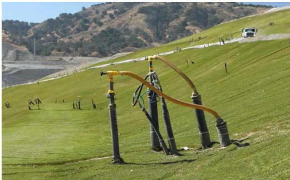
**SYLMAR, Calif. (July 27, 2018)** – As we began reporting last year, the Sunshine Canyon Landfill team has made significant enhancements to our landfill gas collection and control system. In 2017, we added or replaced 153 gas wells and installed 253 pumps to remove trapped leachate from the wells and ensure proper gas well operation.
