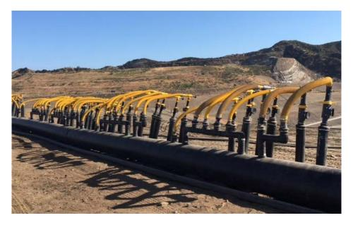
**SYLMAR, Calif. (July 6, 2018)** – Since early 2017, the Sunshine Canyon Landfill team has made enhancements to our landfill gas infrastructure to more effectively collect and control landfill gas. One of the enhancements we've implemented – a remoted wellhead – is a series of multiple wellheads affixed to a common location where vacuum is applied to pull landfill gas from the Landfill. This system provides multiple benefits, including:
