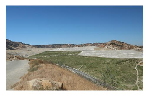
**SYLMAR, Calif. (June 15, 2018)** – In 2017, the Sunshine Canyon Landfill team installed closure turf – an impermeable synthetic liner overlain by artificial turf – over 21 acres of the Landfill to support landfill gas collection and control efforts. As an enhanced landfill cover, closure turf helps prevent landfill gas from escaping and reinforces landfill gas system enhancements we've made at the site.
