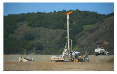
**SYLMAR, Calif. (May 18, 2018)** – Since the beginning of 2018, the Sunshine Canyon Landfill team has continued installation of landfill gas well infrastructure, as we work to expand and optimize our landfill gas system. So far, 49 of the 52 planned gas wells have been installed. The remaining three will be installed by June 1. We will keep you updated as we make further progress on this project.
