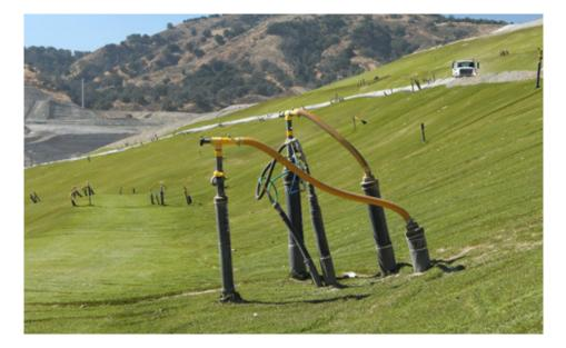
**SYLMAR, Calif. (March 16, 2018)** – In January, the Sunshine Canyon Landfill team began installing 26 new landfill gas wells, as we continue to optimize and expand our landfill gas system. This week we passed the halfway mark and installed the 14th gas well of this project. An additional drill rig will soon arrive on-site to help accelerate this work.
