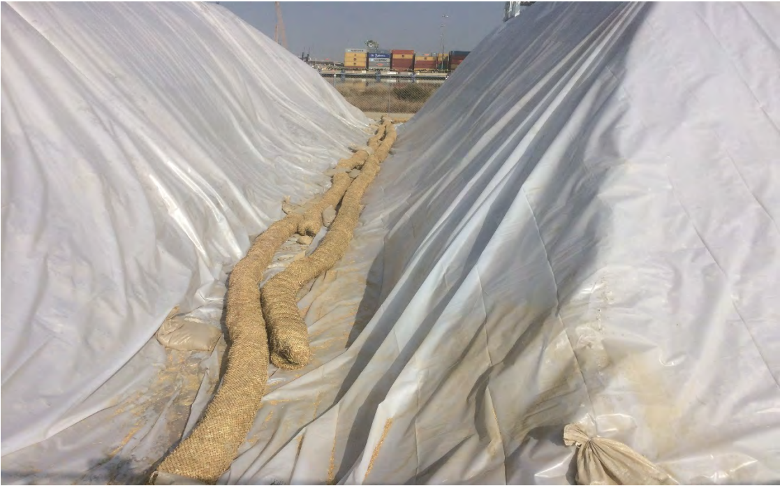
Viewing N between covered stockpiles with waddles in place.
