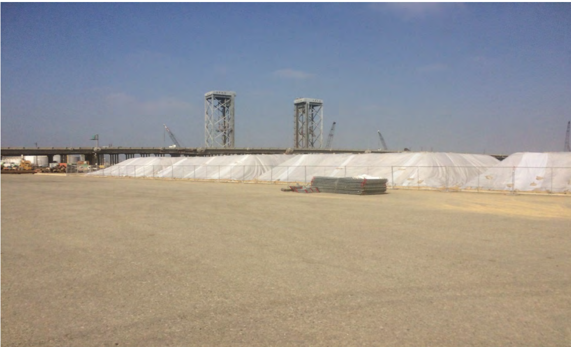
Viewing NW at the final soil stockpiles SP-1 through SP-4.
