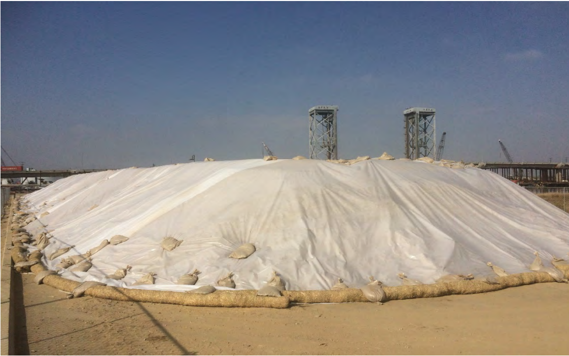
Viewing W at eastern side of completed soil stockpile SP-4.
