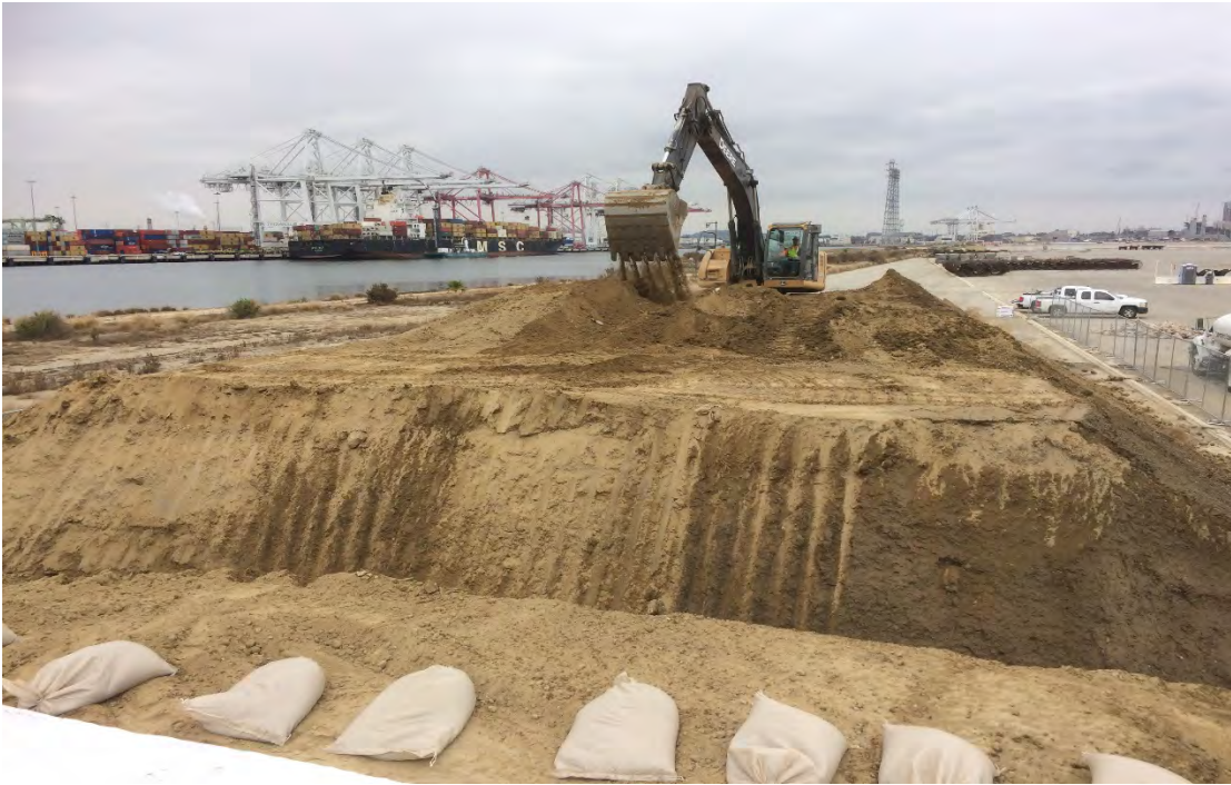
Viewing E at stockpile preparation.
