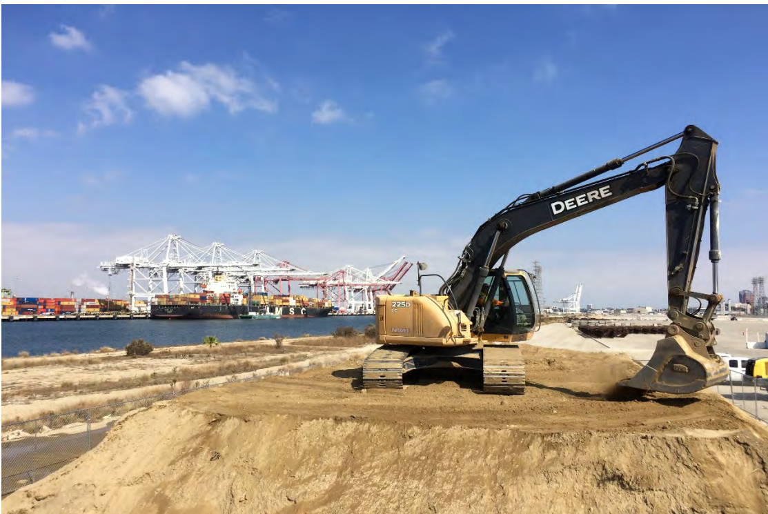
Viewing E at stockpile preparation.
