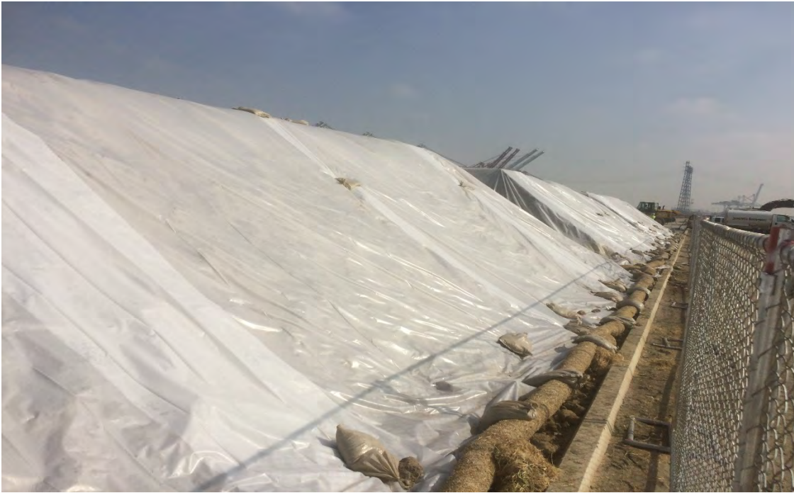
Viewing E at south side final covered soil stockpiles.
