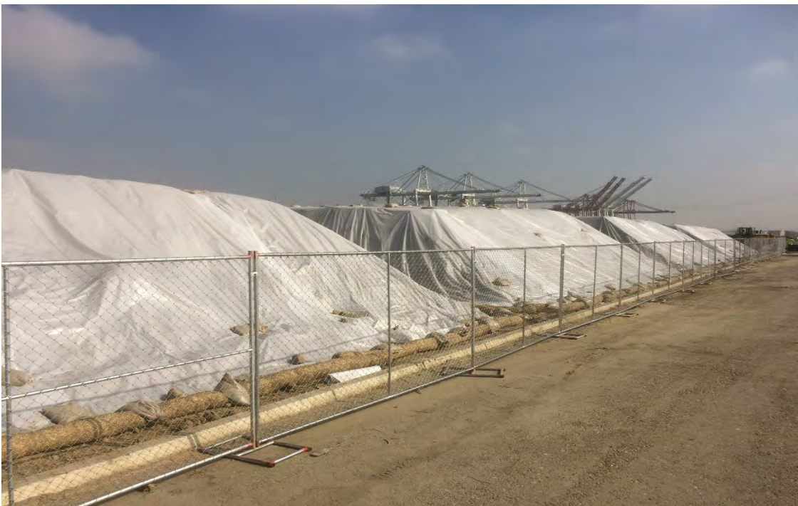
Viewing E at south side final covered soil stockpiles, protected by chain-link fence.
