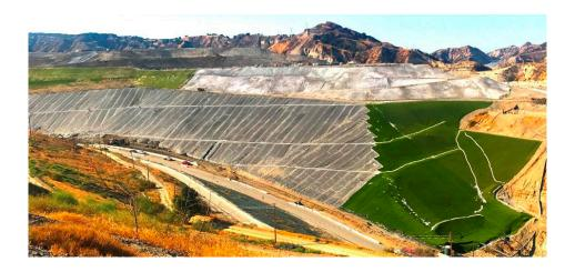
**SYLMAR, CA (Aug. 11, 2017) –** The Sunshine Canyon Landfill team continues to make progress installing closure turf and applying spray-on cover, two of the enhanced landfill covers we are using to prevent landfill gas from escaping. To date we have installed 20 acres of the closure turf primary layer and 10 acres of the final layer. We also applied an additional six acres of spray-on cover this week, raising the total coverage to 33 acres.
