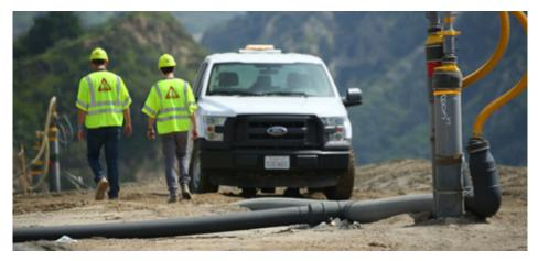
**SYLMAR, CA (June 23, 2017)** – As waste naturally decomposes in a landfill, it creates gas that can be collected and controlled so that it does not migrate off-site. At Sunshine Canyon, we collect landfill gas through a series of pipes and over 800 landfill gas wells to keep landfill gas on-site where it is properly collected and safely managed.
