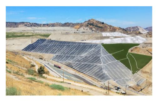
**SYLMAR, CA (July 28, 2017)** – In previous updates, we have reported on progress we have made installing closure turf, one of the multiple enhanced landfill covers to strengthen the effectiveness of the gas collection system. Installation includes two steps – (1) securing the primary closure turf layer, an engineered geomembrane deployed directly on the Landfill's surface, and (2) overlaying the primary layer with a synthetic turf.
