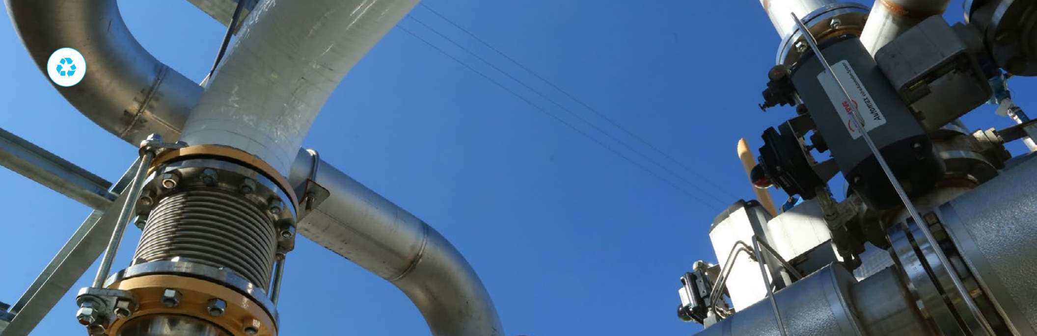
Landfill gas-to-energy infrastructure at Sunshine Canyon Landfill – Sylmar, CA
