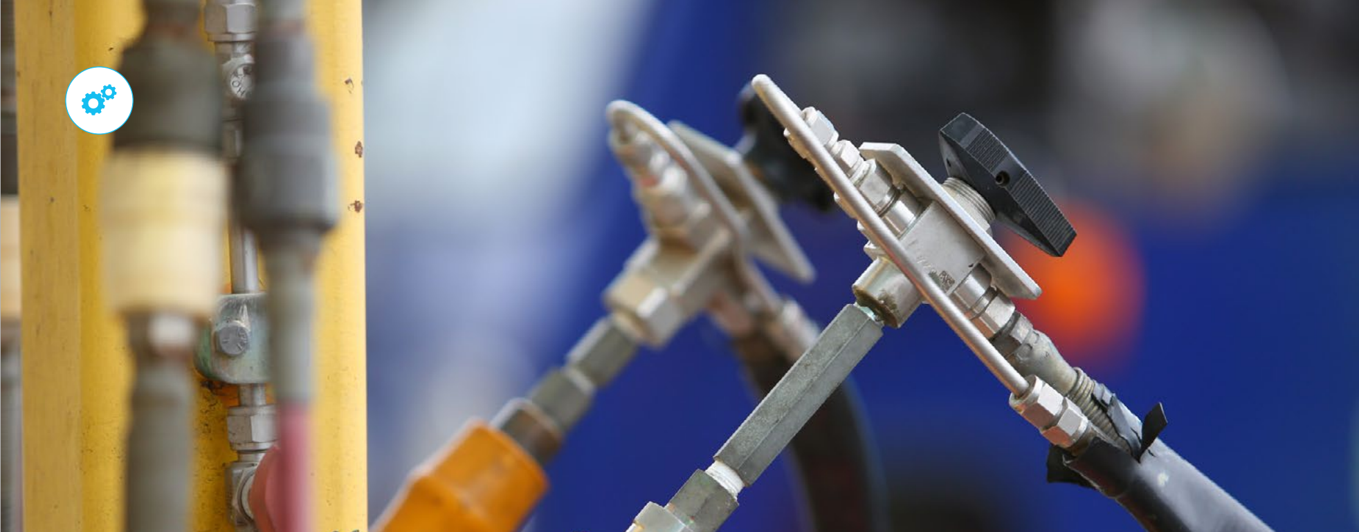
CNG fueling station equipment – Gardena, CA
