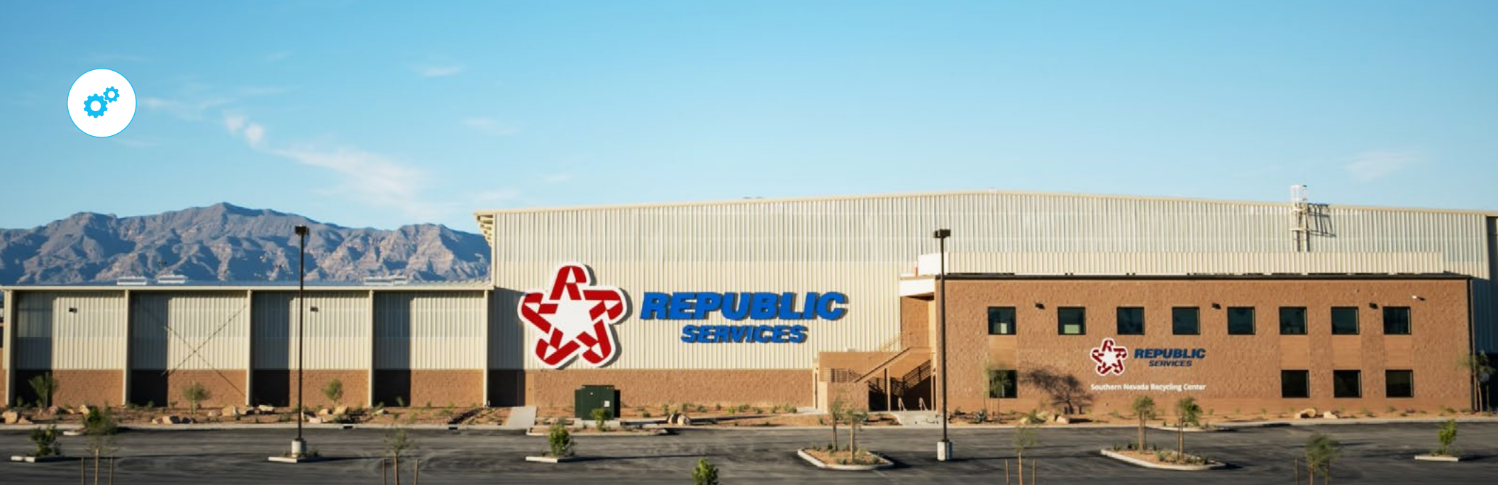
Southern Nevada Recycling Center – North Las Vegas, NV
