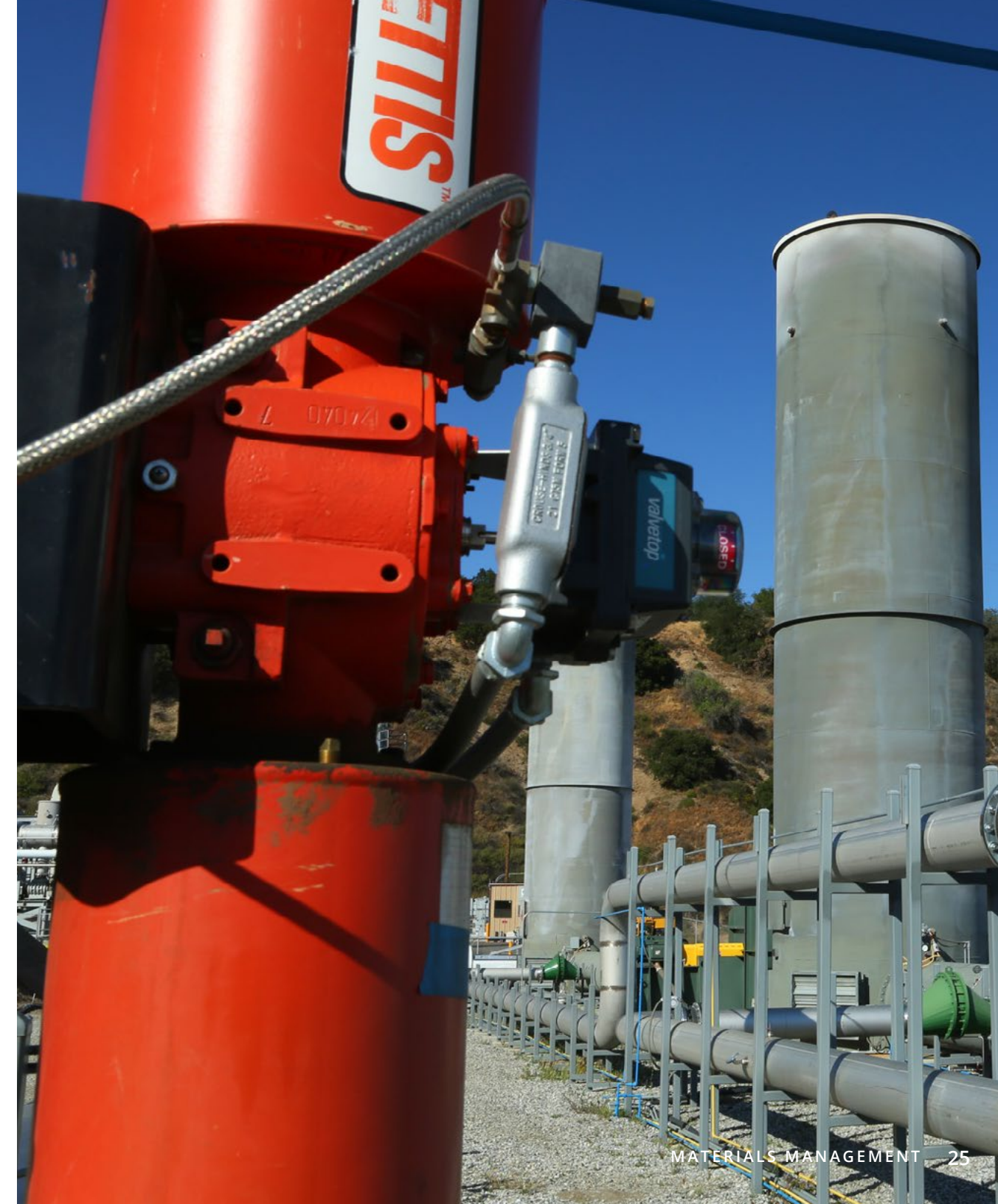
Landfill gas-to-energy infrastructure at Sunshine Canyon Landfill – Sylmar, CA
