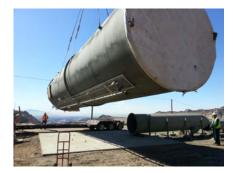
Landfill gas is drawn through the system by way of a 300 HP gas blower; a 250 HP air combustion blower provides excess air and helps achieve an optimum fuel mixture before the gas is flared. With the addition of Flare 10, the facility is now capable of handling up to 22,500 cubic feet per minute of landfill gas.
